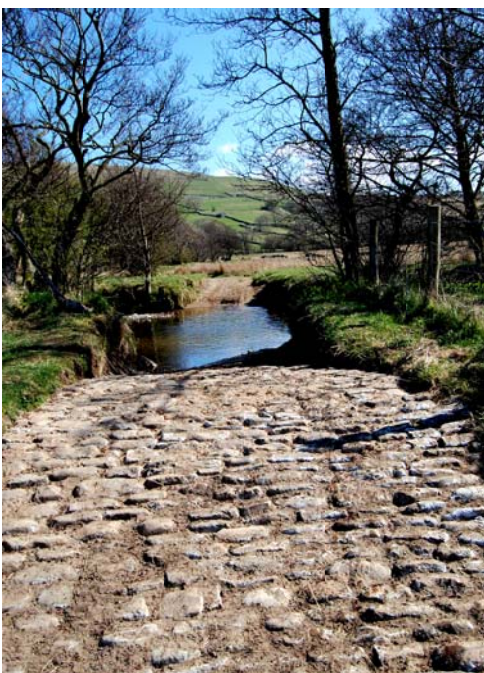
The repaired Raydale track
