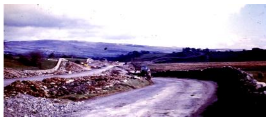
Notice how the walls beside the new straightened road, still visible, go up and down over the hillocks. That practice was ended later.
