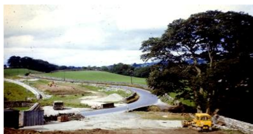
Towards Hawes, work in progress
